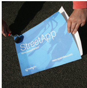
Remove the release liner in small sections at a time and continue to apply - don't be tempted to remove all the liner at once!
