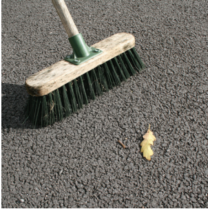
Before application remove loose dirt from the surface with a stiff brush.
