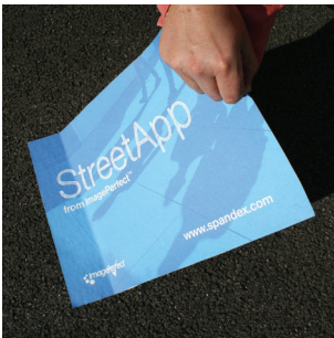
Remove the release liner in small sections at a time and continue to apply - don't be tempted to remove all the liner at once!
