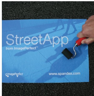
Roll the film again with either a rubber roller, such as that pictured, or with the RollePro soft application roller (below) which will facilitate the bond of the product to the structured surface. Roll slowly several times to achieve firm adhesive contact. For larger applications, a wide roller is recommended.
