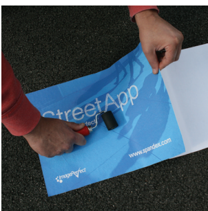
Roll the film again with either a rubber roller, such as that pictured, or with the RollePro soft application roller (below) which will facilitate the bond of the product to the structured surface. Roll slowly several times to achieve firm adhesive contact. For larger applications, a wide roller is recommended.
